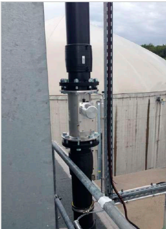
Installation of the GD 300 in a vertically falling line
