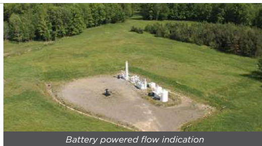
Battery powered flow indication
